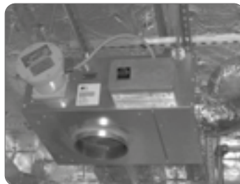
B-MARINE: with ATEX heater
